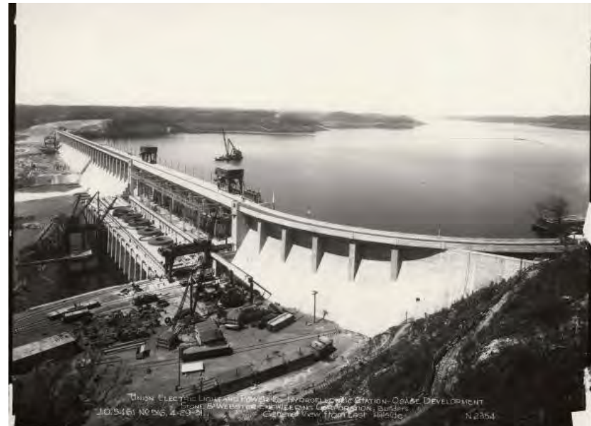
Bagnell Dam 1931, Source: Missouri State Archives
