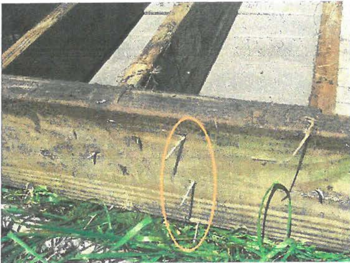
Figure 1. Close-up of deck ledger that was connected to a structure with nails only. When lightly loaded by occupants, the deck shifted laterally, pulling the nails out of the supporting structure.
